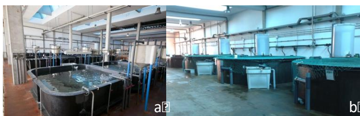
Figure 9.3.2. a) Tanks of 10 \text{ m}^3 at P2. FCPCT facilities, b) 40 \text{ m}^3 tanks
