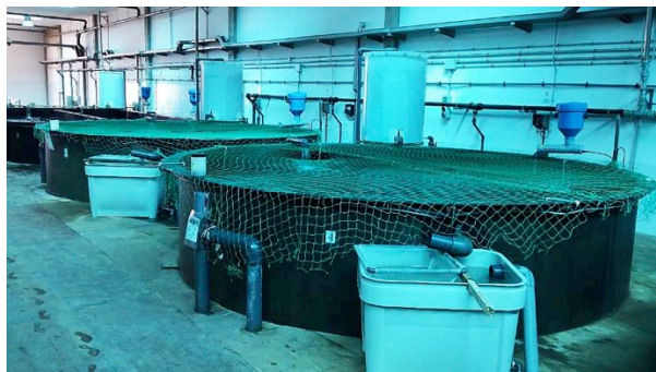
Figure 9.3.2. Set of tanks of 40 m 3 for greater amberjack broodstock at FCPCT facilities.
