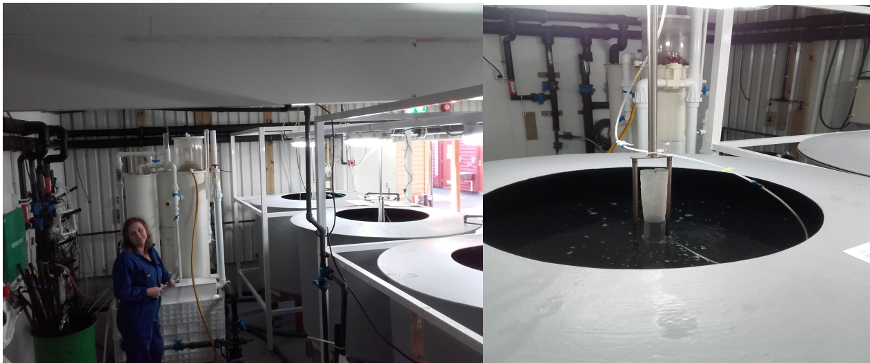
Figure 17.3.3. First feeding tanks attached to the RAS system.
