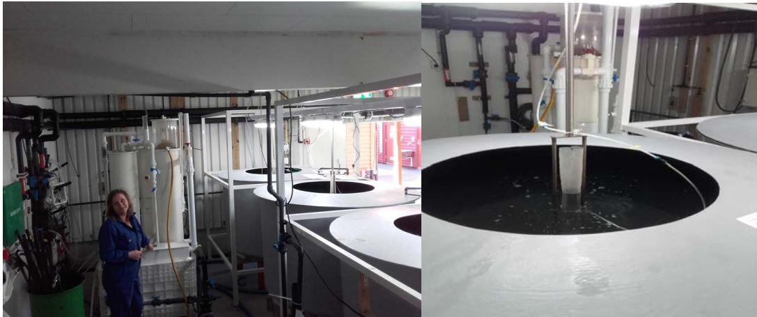
Figure 17.2.6. First feeding tanks attached the RAS system.
